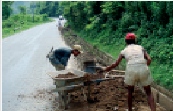
Routine maintenance by Lengthworkers
