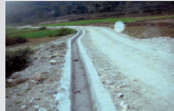
Maintenance of side drain at Syangja
