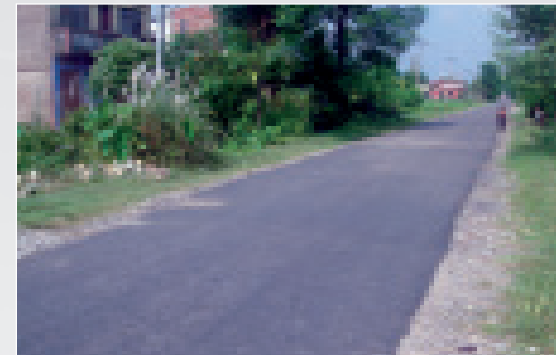
Road surface maintained through Ottaseal
