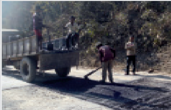
Patchwork -Recurrent Maintenance
