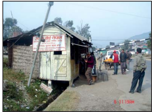
Toll Collection Booth Narayanghat-Butwal Road Section
