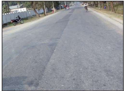
Well Maintain Road in Pokhara Submetropolitan
