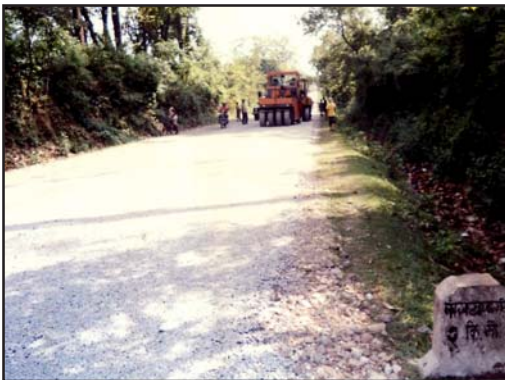
Preparation for Maintain Reseciling work
