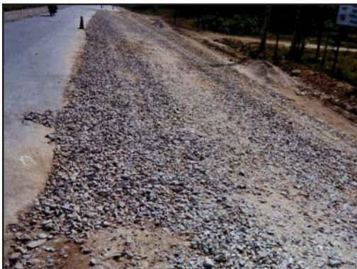
Repar of the Pavement (Spot Maintainmance)
