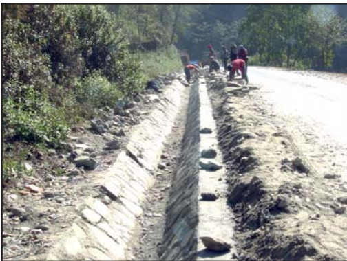
Repair of Side Drain
